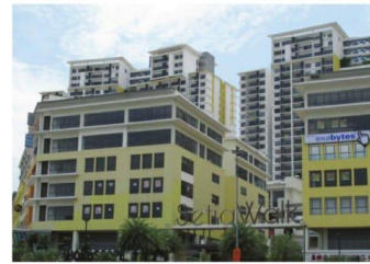
完成后的抹灰工程，品质优越。 Project completed with excellent quality.
